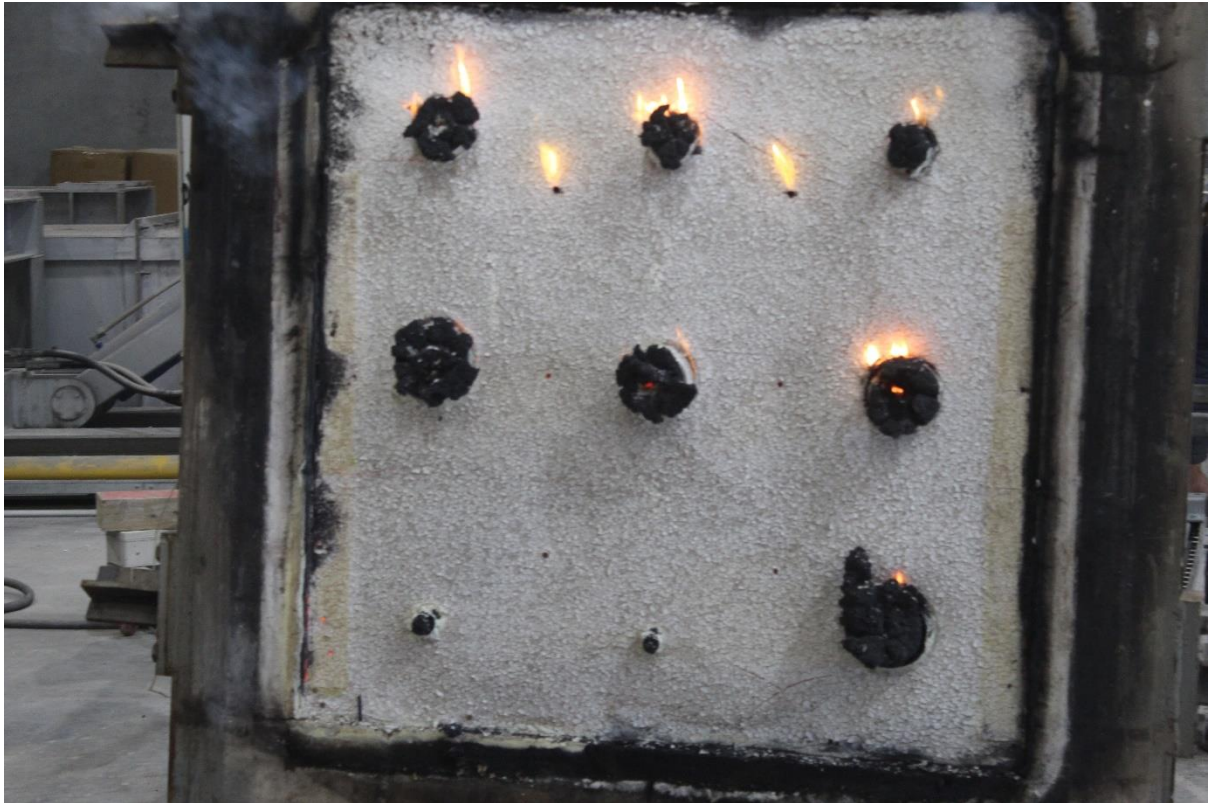
Figure 21 – Exposed face after the test
